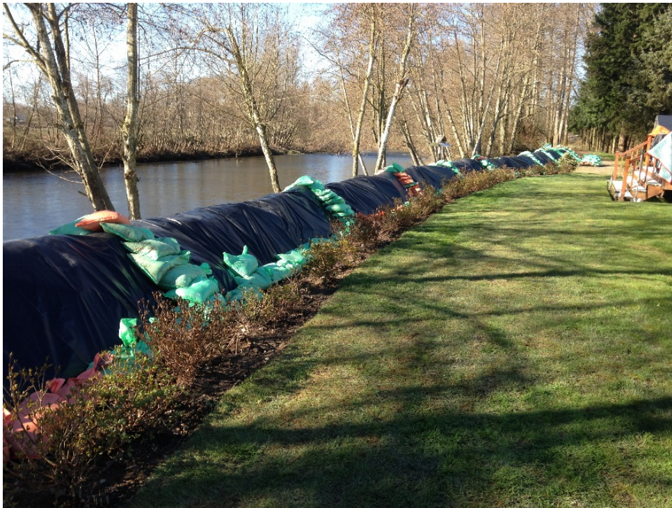
Figure 11: Sand bag berm installed along top of levee as an interim flood risk reduction measure
