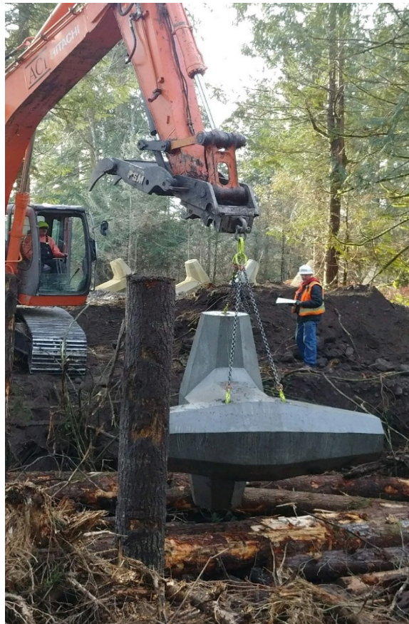
Figure 21: Crews installing an engineered log jam along the Puyallup River in December 2017
