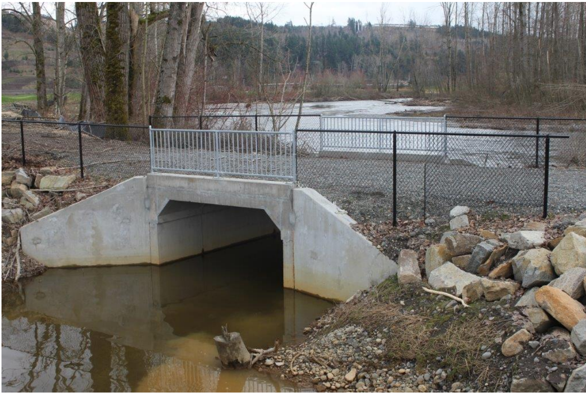
Figure 1: FHPA #20; Image of the completed culvert that was installed by the City of Sumner.
