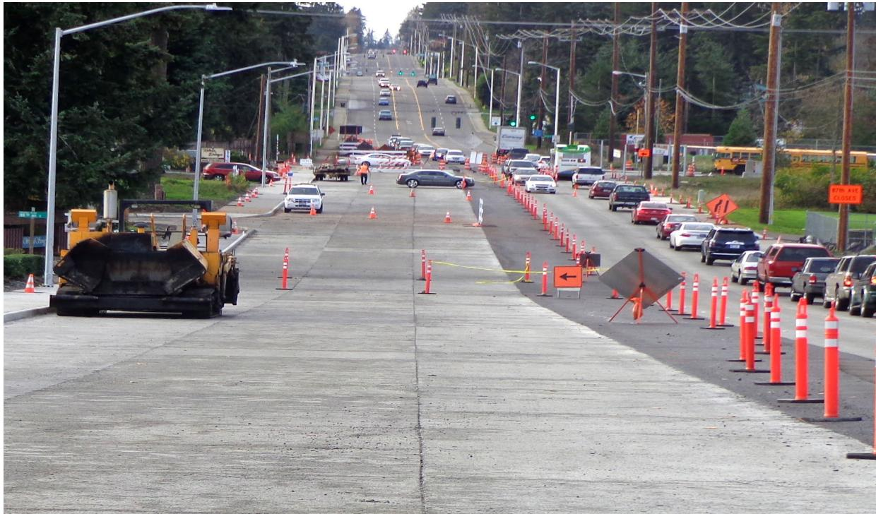
In 2015, the City of Puyallup used a portion of their Opportunity Funds to install pervious concrete sidewalks and roadways along 39th Avenue SW and 11th Street SW to 17th Street SW. The City also installed new lights and signals along this roadway and improved other necessary infrastructure in the area.
