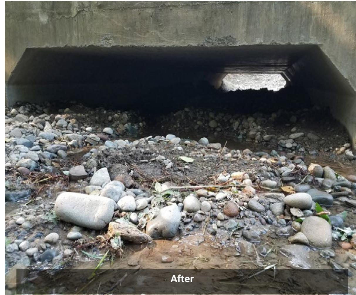
In 2017, the City of Edgewood requested to use a portion of their Opportunity Funds for the Jovita Boulevard Box Culvert Maintenance Project. This project removed 20 cubic yards of sediment and outwash material that allows for minor culvert repairs. Completion of this project will assist with year-round positive drainage through an existing box culvert.
